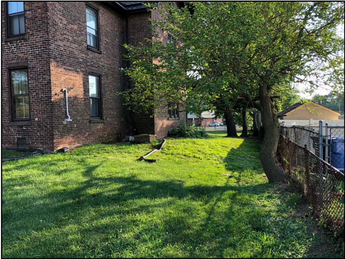
Plate 6.4: View of the rear (north) yard of the Dunham House. View: West. Photographer: Michael J. Gall, July 10, 2019.
