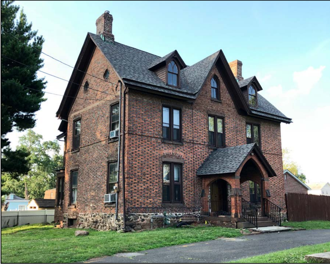
Plate 6.1: View of the front (south) and west sides of the Dunham House. View: Northeast. Photographer: Michael J. Gall, July 10, 2019
