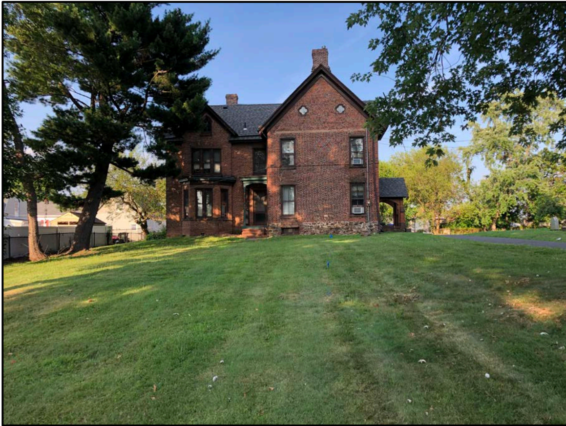
Plate 6.2: View of the west side yard of the Dunham House showing the west façade. View: East. Photographer: Michael J. Gall, July 10, 2019
