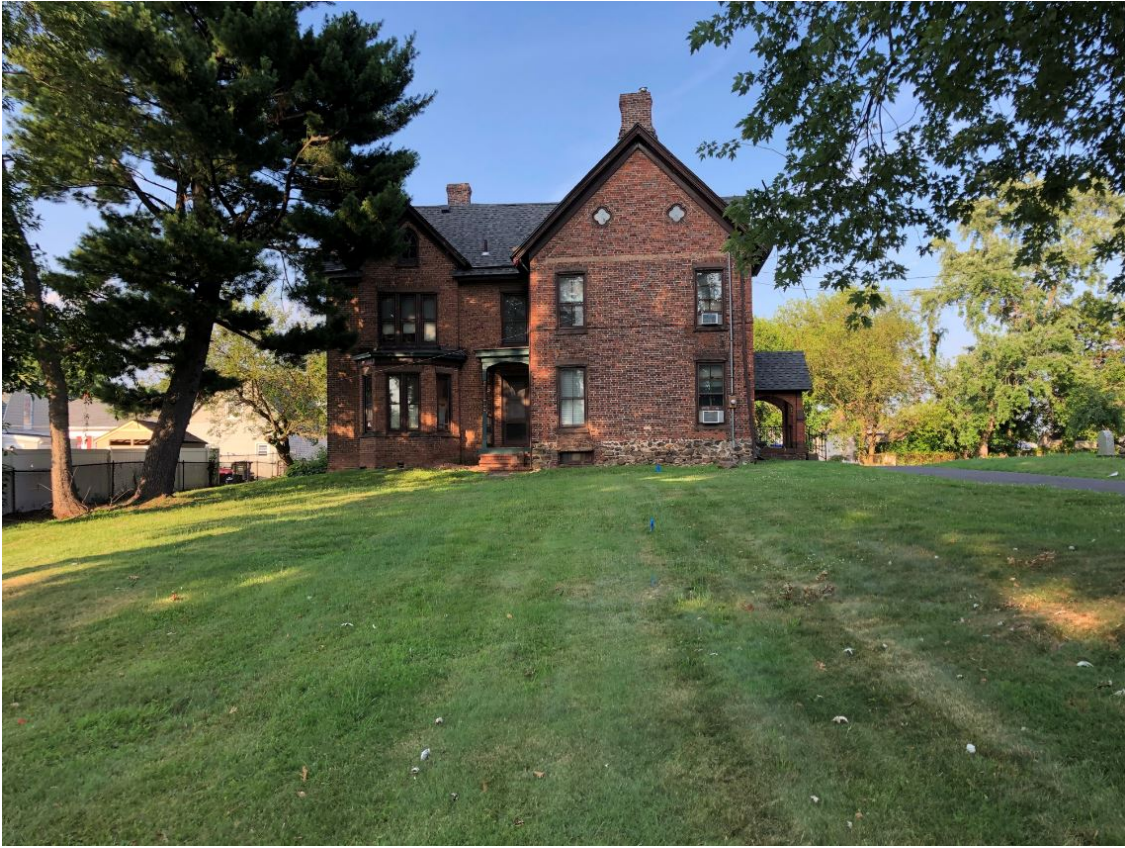
Plate 2: View east showing the side yard of the Jonathan Dunham house (current Rectory), July 10, 2019
