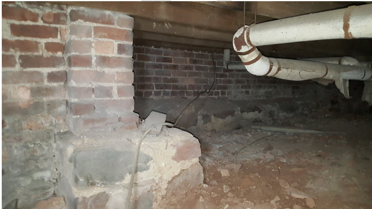
Figure 5: View of the crawl space under the rear addition looking east. The lower courses are all of stone. Photograph by Mark Nonestied
