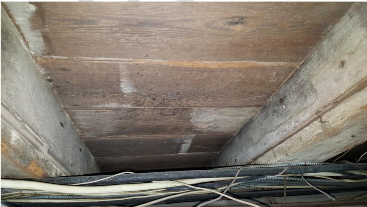
Figure 4: View of the recycled flooring showing the reciprocating saw marks. Photograph by Mark Nonestied
