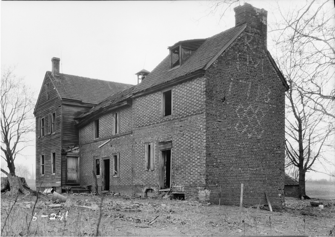
Figure 4.4: John Rogers House, Springside, Burlington County, c. 1718. Note the panel of four diamonds on the wall, beneath the date 1718 and the initials IRM (HABS NJ 241).
