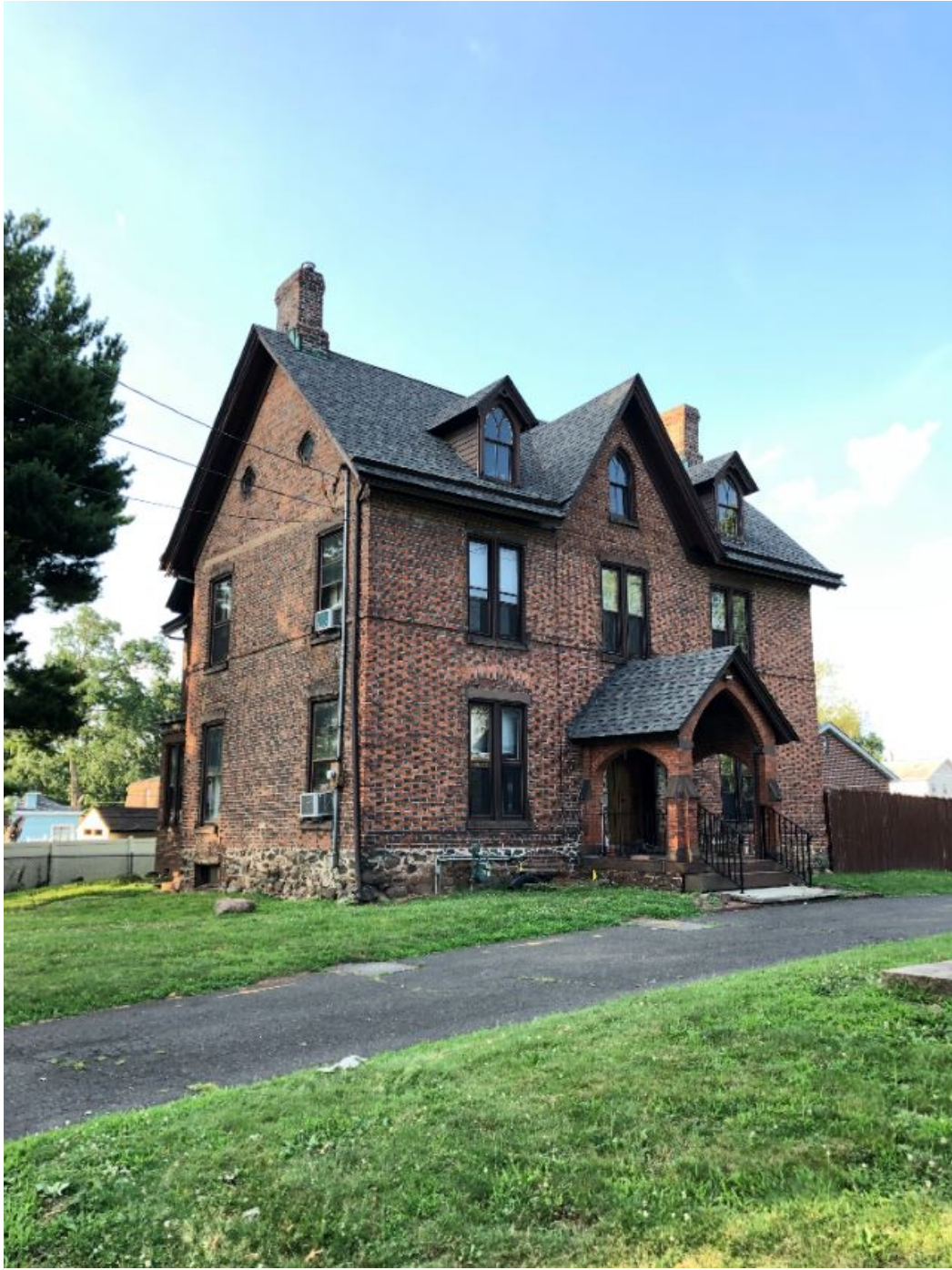
Plate 1: View northeast of the Jonathan Dunham house (current Rectory), July 10, 2019
